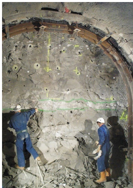
Fig. 2.1 Heterogeneous distribution of carbonates (light grey) in the COX carbonate-rich unit observed in a drift at the -445 m level of the URL Bure (Andra)
