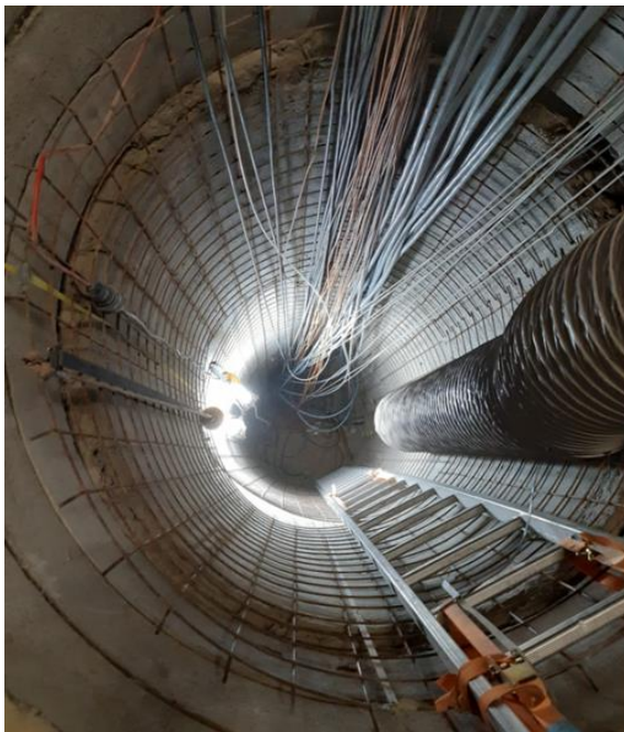
Fig. 3.42 View of the Shaft 1 during installation phase
