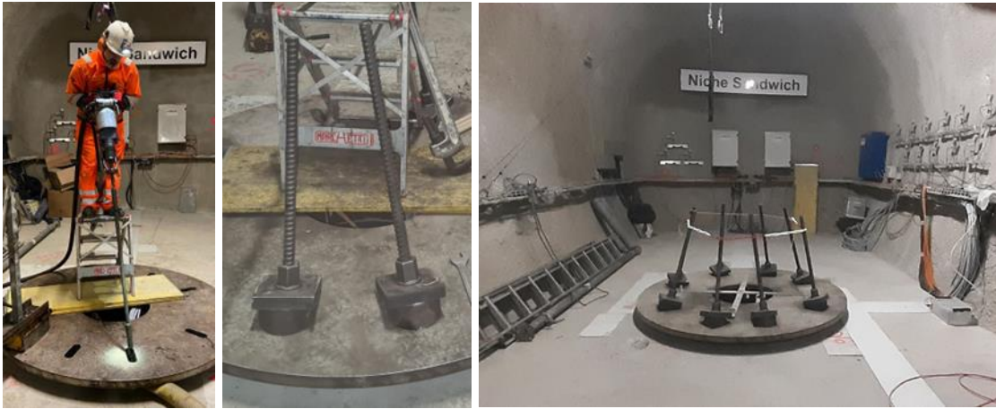
Fig. 3.61 Bolting of the top lid for Shaft 1
