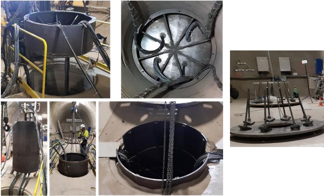
Fig. 3.92 Installation of the confining tube and the closure lid for Shaft 2
