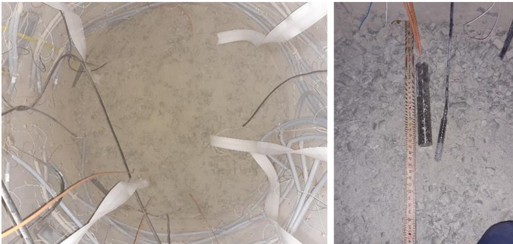
Fig. 3.49 Installation of DS1 in Shaft 1
