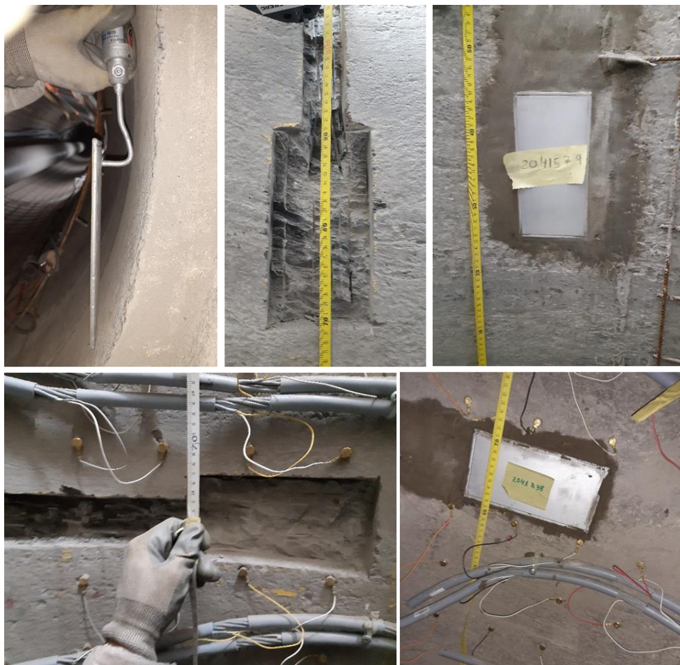
Fig. 3.47 Installation of radial stress sensors at the wall of Shaft 1
