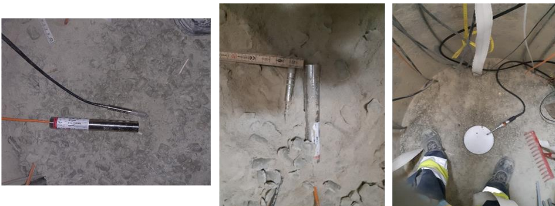
Fig. 3.54 Installation of DS3 in Shaft 1
