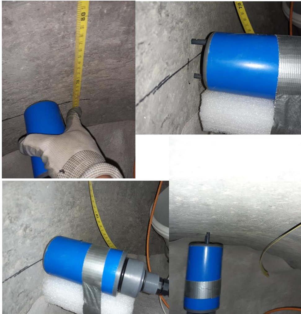
Fig. 3.45 Installation of twin rod TDR sensors in Shaft 1
