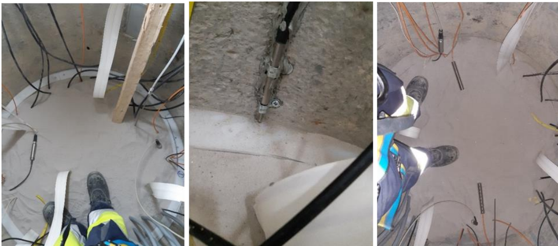
Fig. 3.53 Installation of displacement measurement system on top of ES3 in Shaft 1
