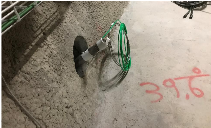
Fig. 3.14 Feeding borehole BSW-B25 with steel casing
