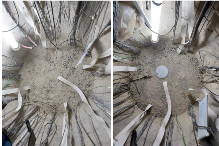
Fig. 3.87 Installation of DS3 in Shaft 2
