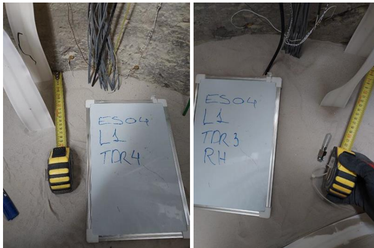
Fig. 3.88 Check of TDR positions during installation of ES4 in Shaft 2
