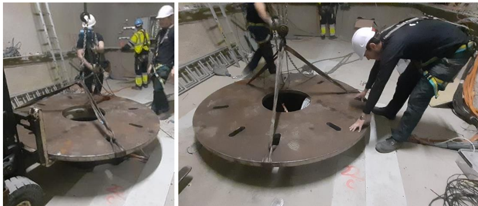
Fig. 3.60 Installation of the top lid for Shaft 1
