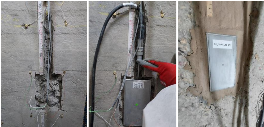
Fig. 3.80 Installation of radial stress sensors at the wall of Shaft 2
