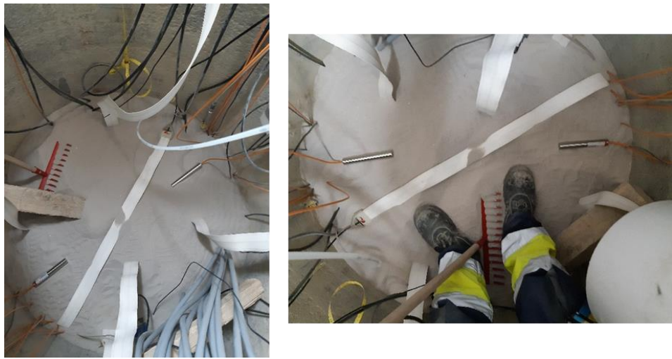
Fig. 3.55 Installation of ES4 in Shaft 1
