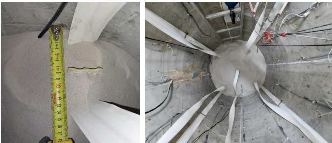
Fig. 3.82 Installation of ES1 in Shaft 2
