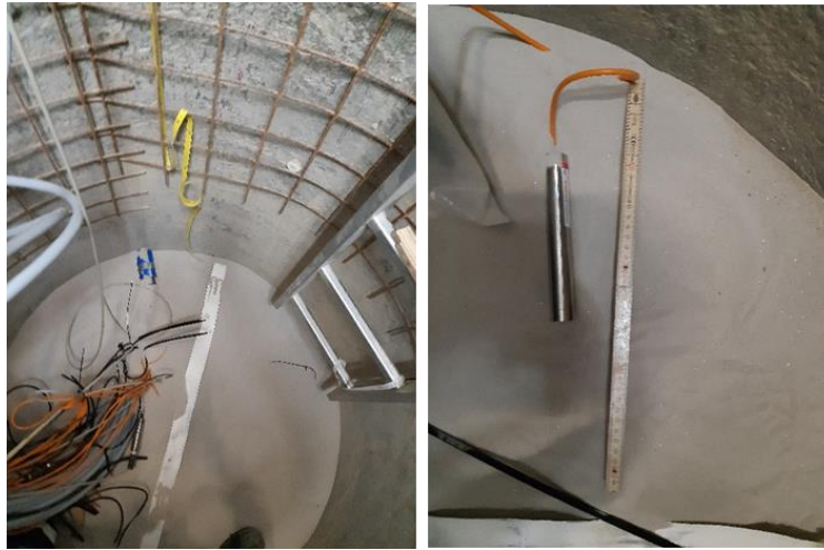
Fig. 3.57 Installation of ES5 in Shaft 1
