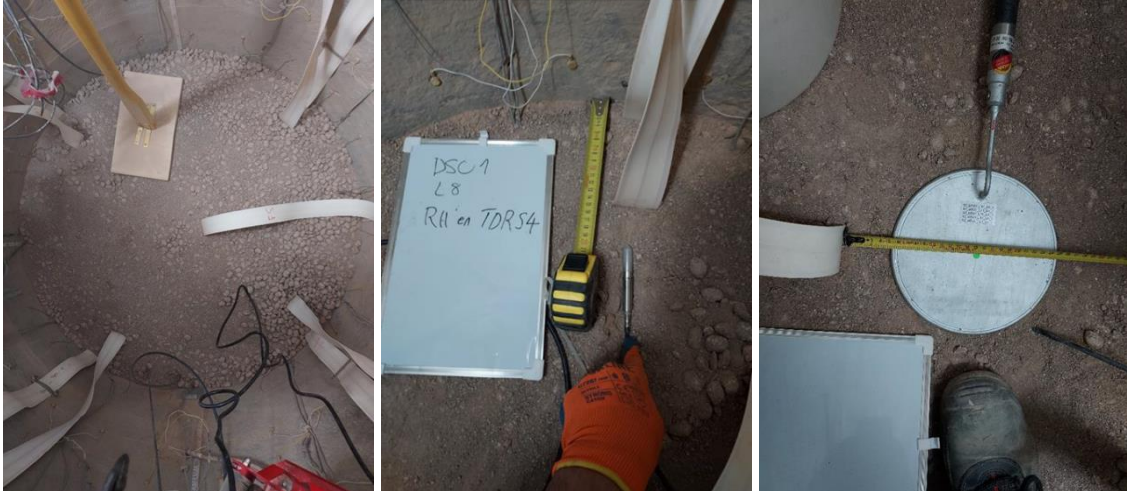
Fig. 3.83 Installation of DS1 in Shaft 2
