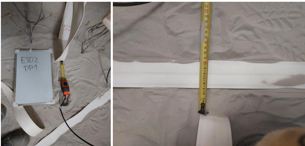
Fig. 3.84 Installation of ES2 in Shaft 2
