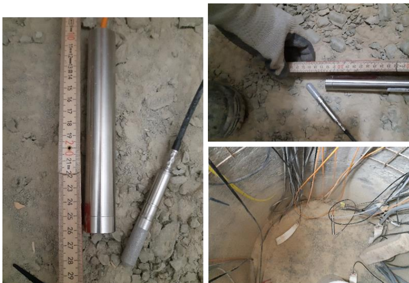
Fig. 3.56 Installation of DS4 in Shaft 1
