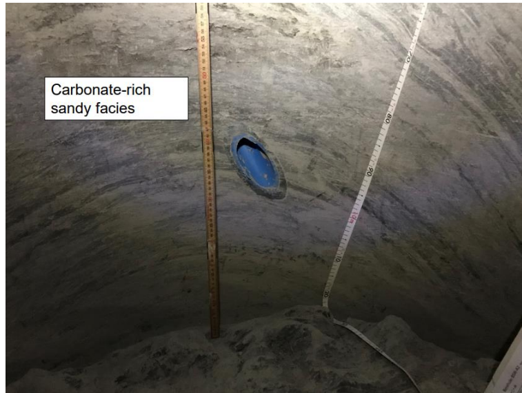
Fig. 3.21 Lowermost part of Shaft 2 in carbonate-rich sandy facies and with outlet of feeding borehole (Photo by D. Jaeggi, swisstopo)
