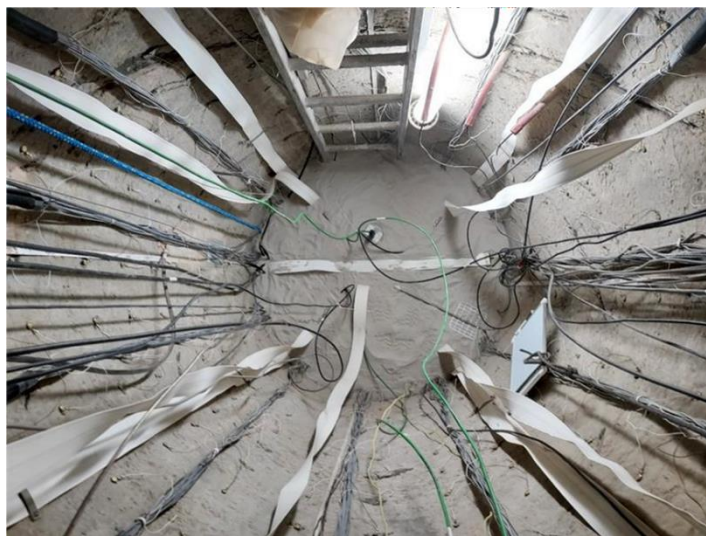
Fig. 3.86 Installation of ES3 in Shaft 2 including one back-up hydration tube
