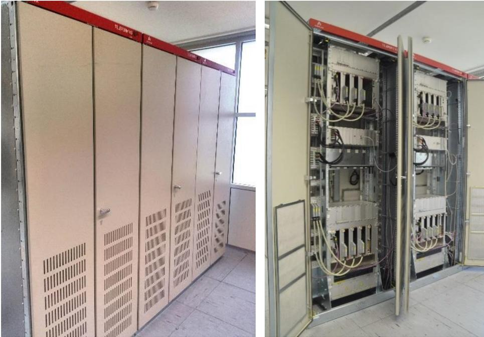
**Figure 1.2** The AnTeS-SIC-real module, a real safety I&C system based on Teleperm XS
