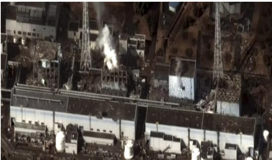
Photo of the Fukushima Daiichi plant, Units 1-4 (from right to left) of 16-03-2011
