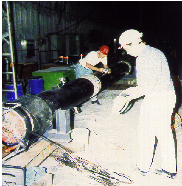
Figure 2-5 DEBORA 1; borehole liner equipped with instruments.
