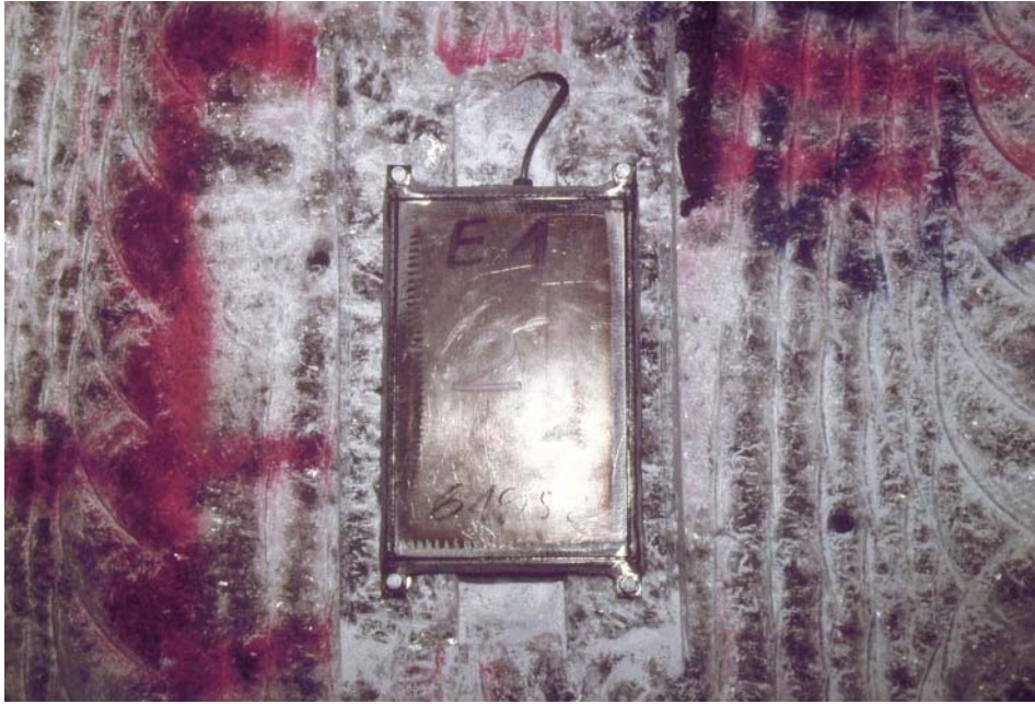
Fig. 5.4.1 Pressure gauge 61975 in situ at the drift wall (bottom side)
