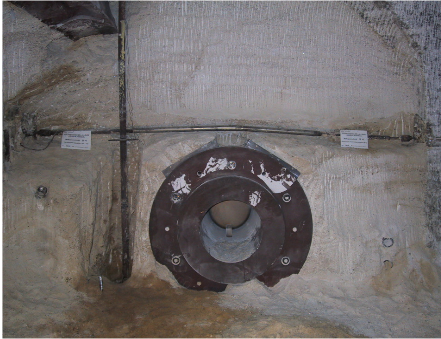
Fig. 5.3.1 Bent horizontal convergence measuring device in situ (cross section B +1 )
