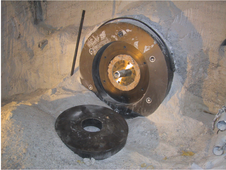
Fig. 3.5 Dismantling of the central heater cask
