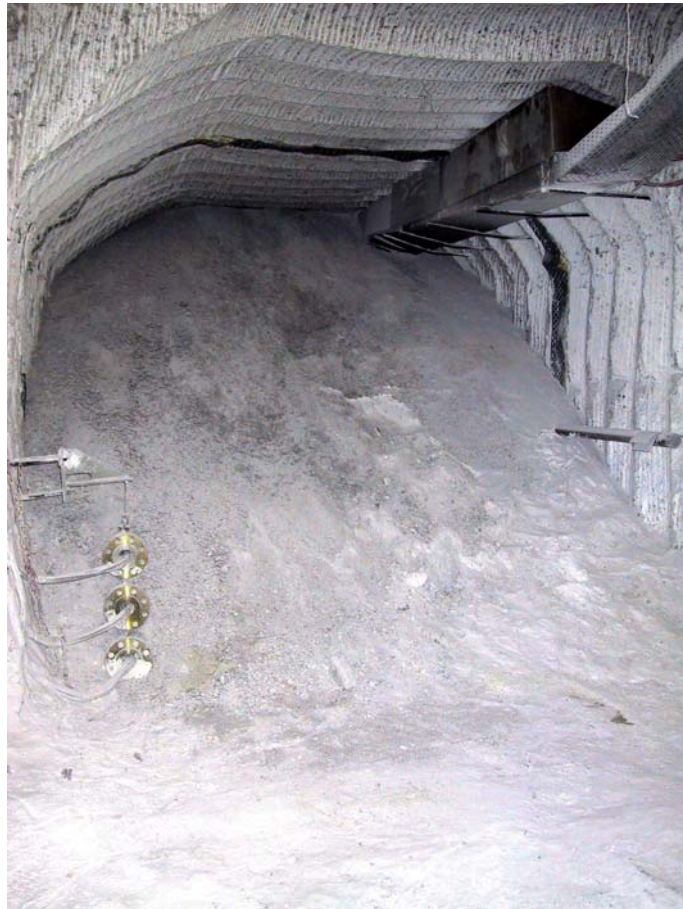
Fig. 4.1.6 Backfill slope at the entrance of drift A
