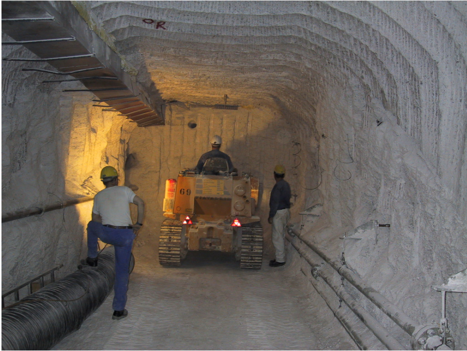
Fig. 3.1 Backfill excavation in the non-heated area using a loader
