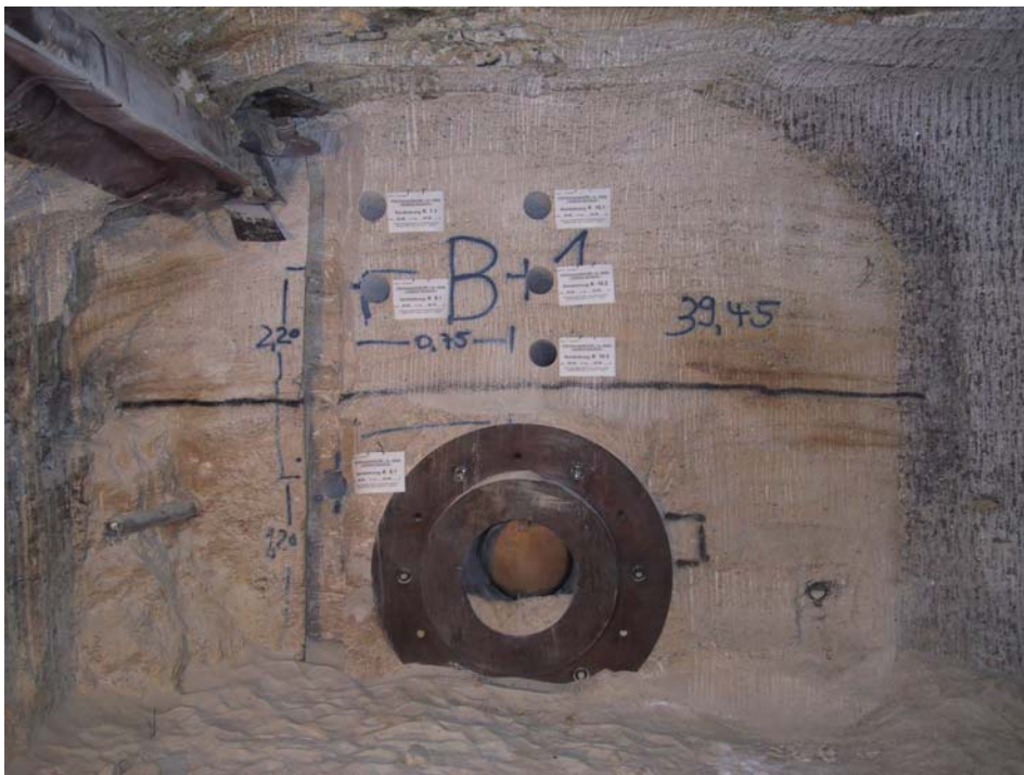
Fig. 3.6 Boreholes and slots in the backfill remaining from sampling at cross section B +1
