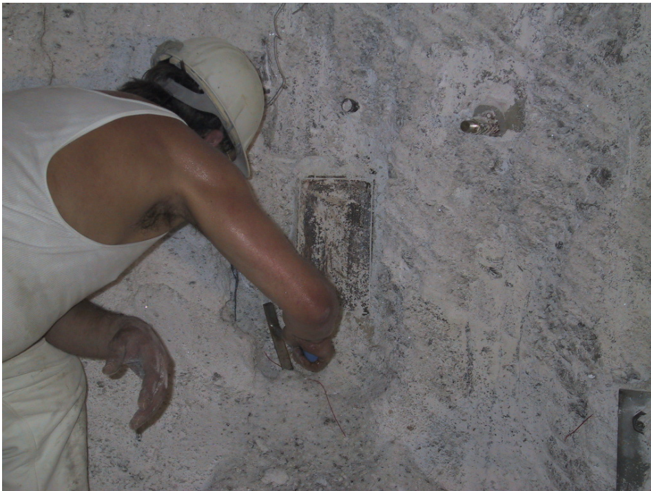
Fig. 3.4 Manual recovery of a hydraulic pressure cell
