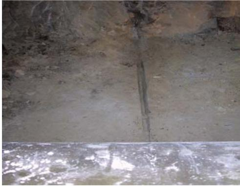
**Figure 3.11a** Completely closed cable slot in the drift wall at cross section D1 of the TSDE test field
