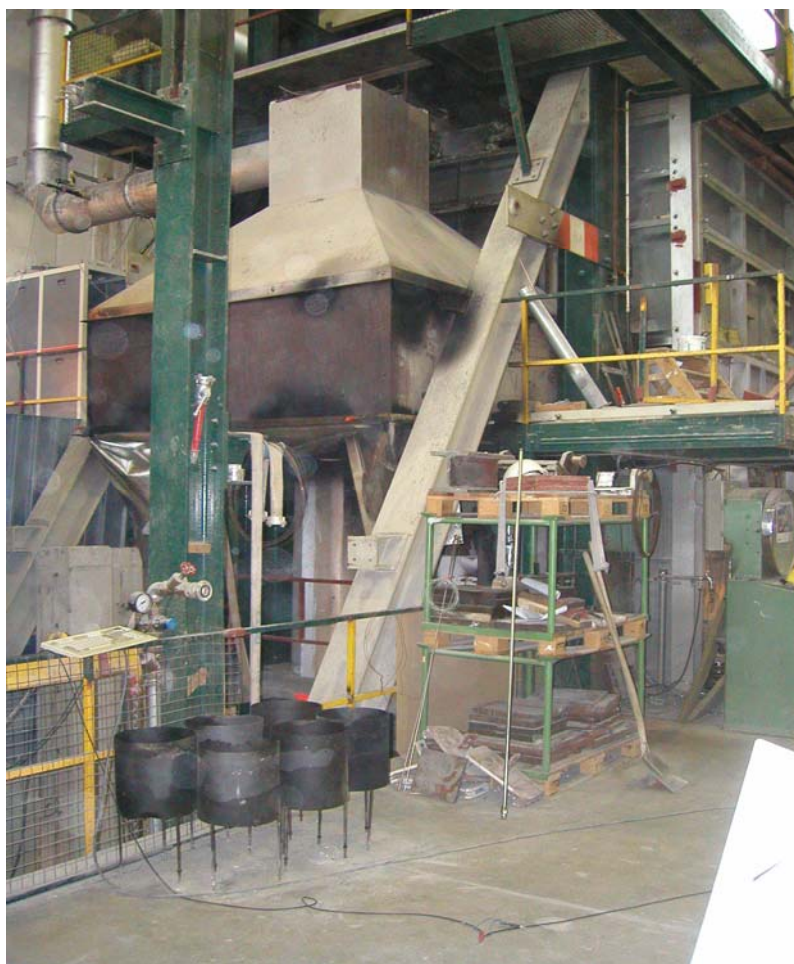
Fig. 2-10 View onto the hood installed above the front door
