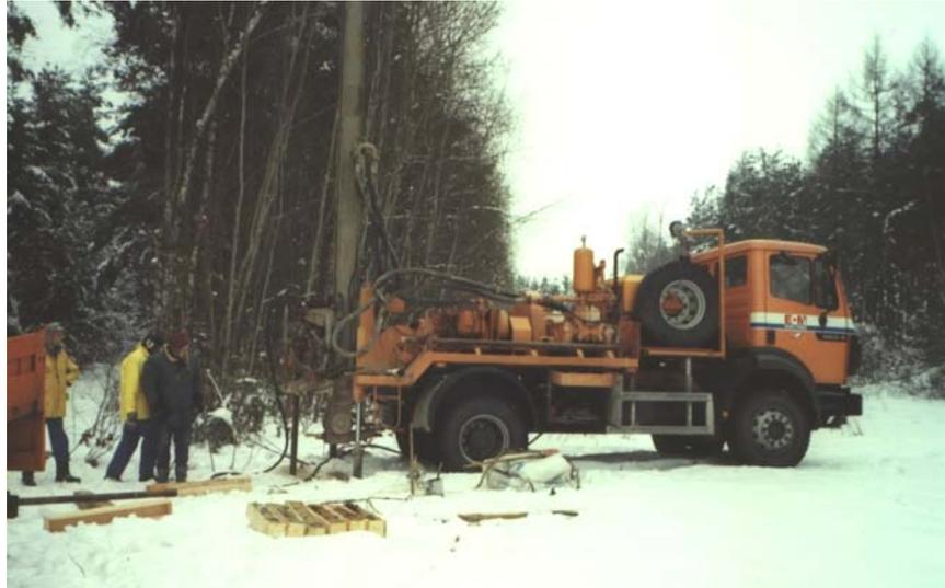
**Fig. 13:** Drilling of well HB02-02 in Keuper sandstone (16.01.2002)
