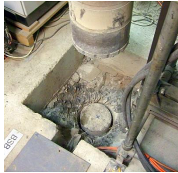
b) Cored concrete plug still in place
