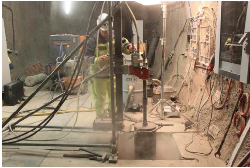
a) Step 1: Coring of a concrete plug
