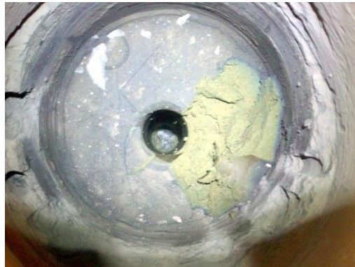
b) Seal with a left core borehole
