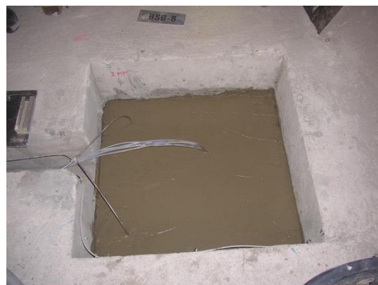
f) Grouted borehole cellar
