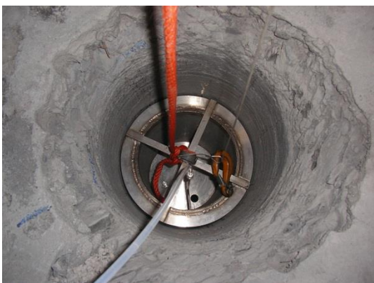
e) Packer in borehole SB2
