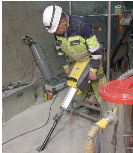
d) Coring of seal material through an inclined borehole
