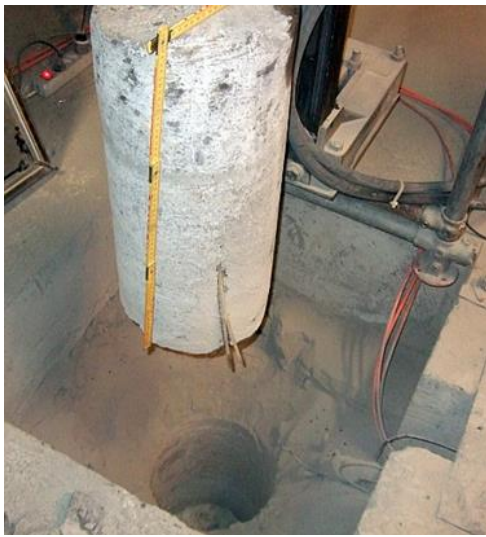
c) Step 2: Retrieval of concrete plug
