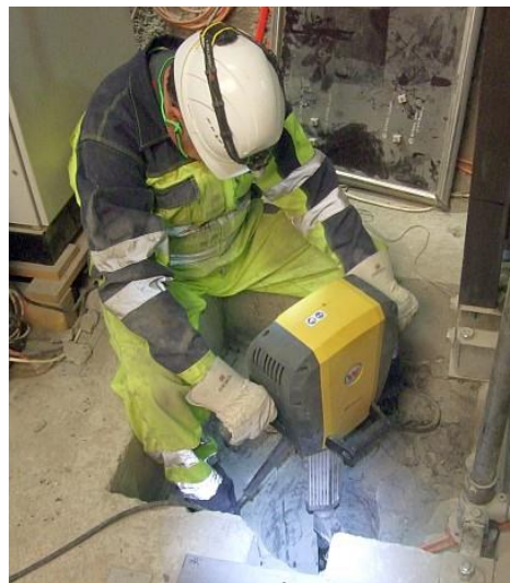
f) Step 4: Coring of seal material
