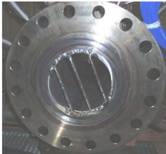
Figure 8: Thermocouples in spool piece flange
