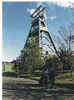
▲ Salzgitter – Konrad repository (in construction)
