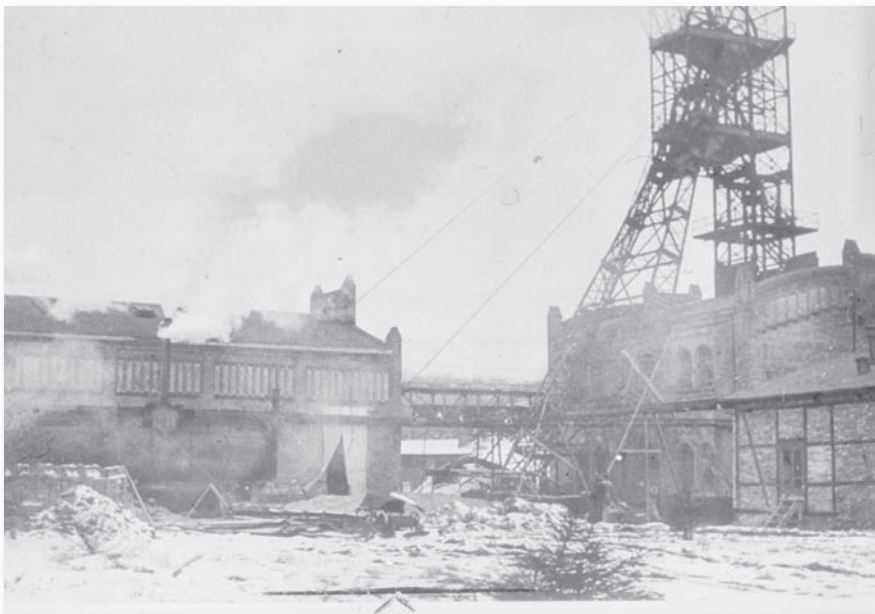
◀ Fig. 3: This photo shows the condition of the aboveground buildings in the year 1964 after the exploitation of the mine was stopped. On the right side you can see the hoist frame on the left side the building for the hoist engine. Both buildings are now listed monuments.
