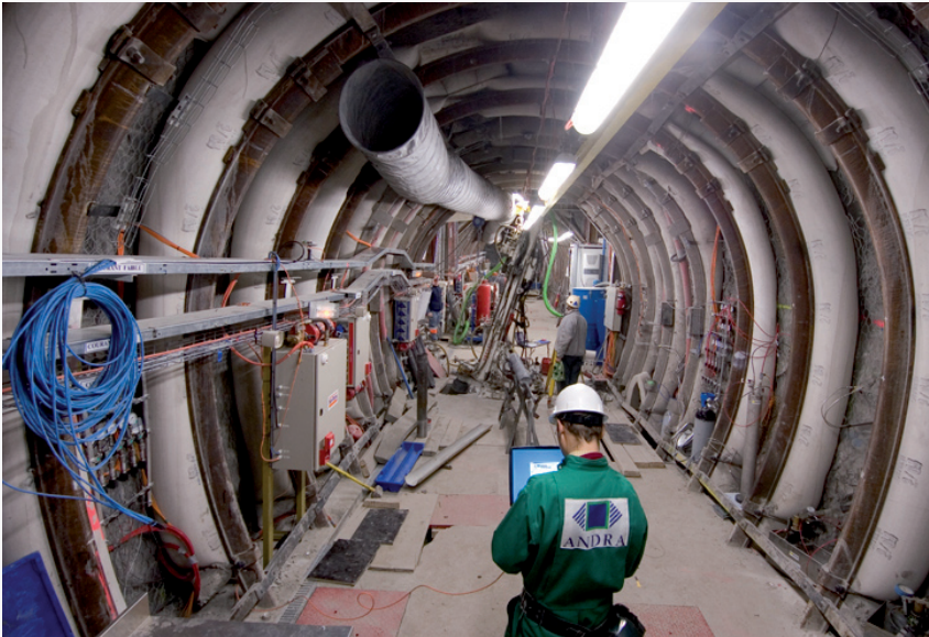
◀ Fig. 2: Experimental drift at a depth of 490 m in the Meuse/Haute-Marne Underground Laboratory.
