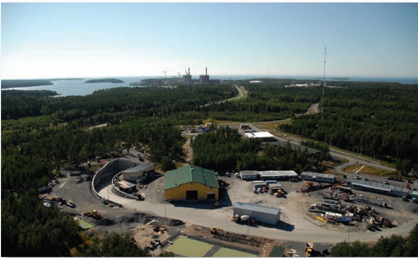
◀ Fig. 2: The location of the ONKALO at Olkiluoto: the mouth of the access tunnel is seen in the foreground.
