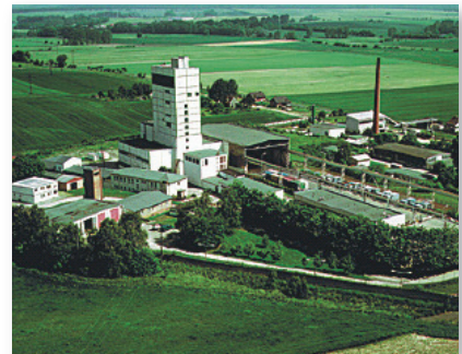
▲ Morsleben – Repository for low and intermediate level radioactive waste (ERAM)
