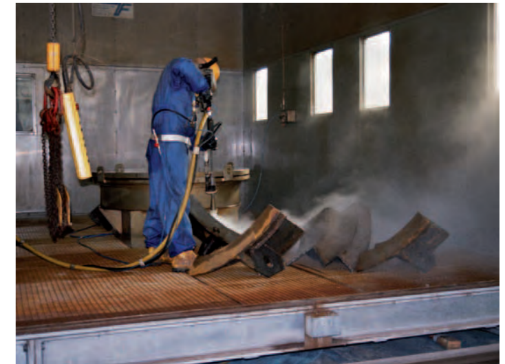
Fig. 26: Decontamination by high-pressure water jet cleaning
