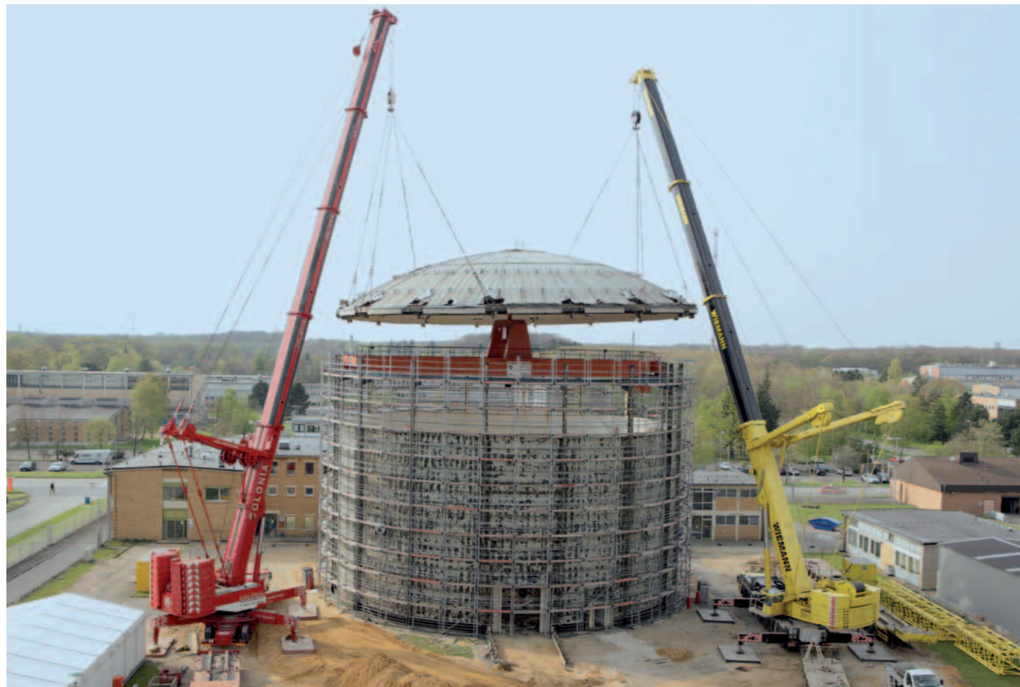
Fig. 6: Dismantling of the FRJ-1 research reactor
