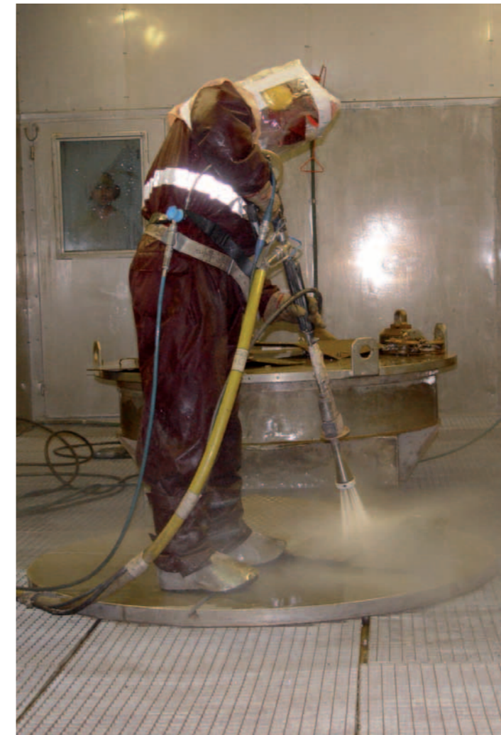
Fig. 24: Full protective clothing during decontamination by high-pressure cleaning
