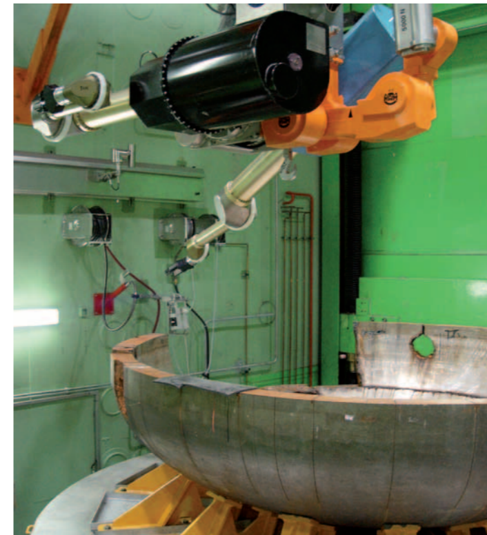
Fig. 29b: Remote-controlled thermal cutting (chamber for dry cutting)
