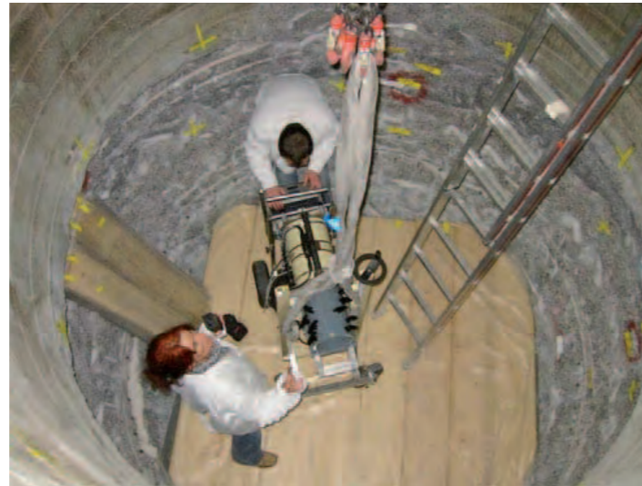
Fig. 7: Control measurements in the reactor cavity of the TRIGA HD II research reactor
