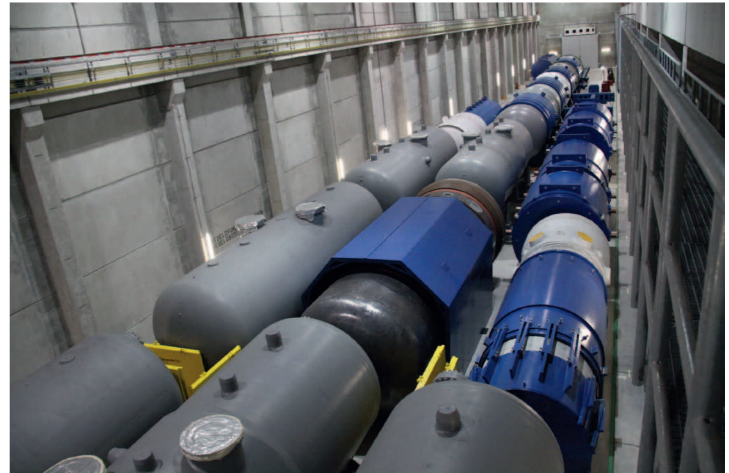
Fig. 42: Decay storage of large components at the Interim Storage Facility North (ZLN)
