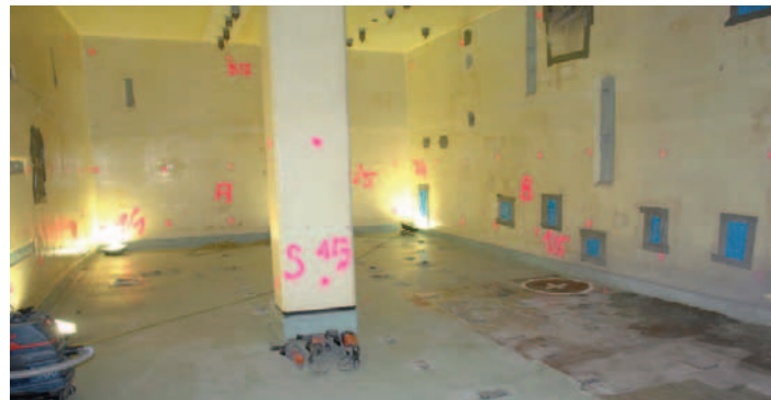
Fig. 35: Room with markings for determining the surface contamination
