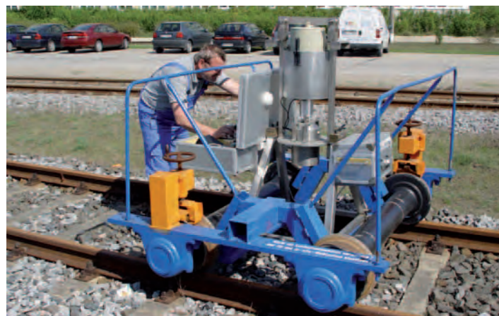
Fig. 36: Measurement for clearance of soil areas
