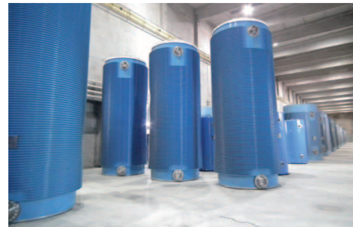
Fig. 40: Transport casks at the Interim Storage Facility North (ZLN)
