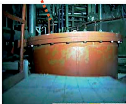
Survey inside the Unit 2's torus (April 18, 2012)
