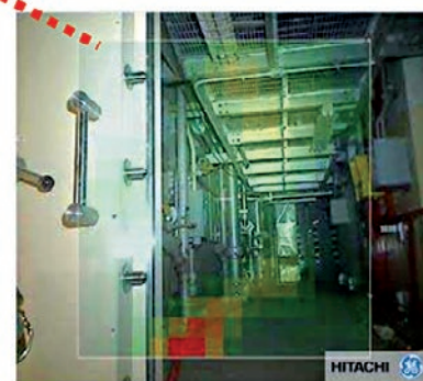
Survey on radiation source and dose rate inside the Unit 1 R/B (photo by gamma camera) (May 14~18, 2012)
