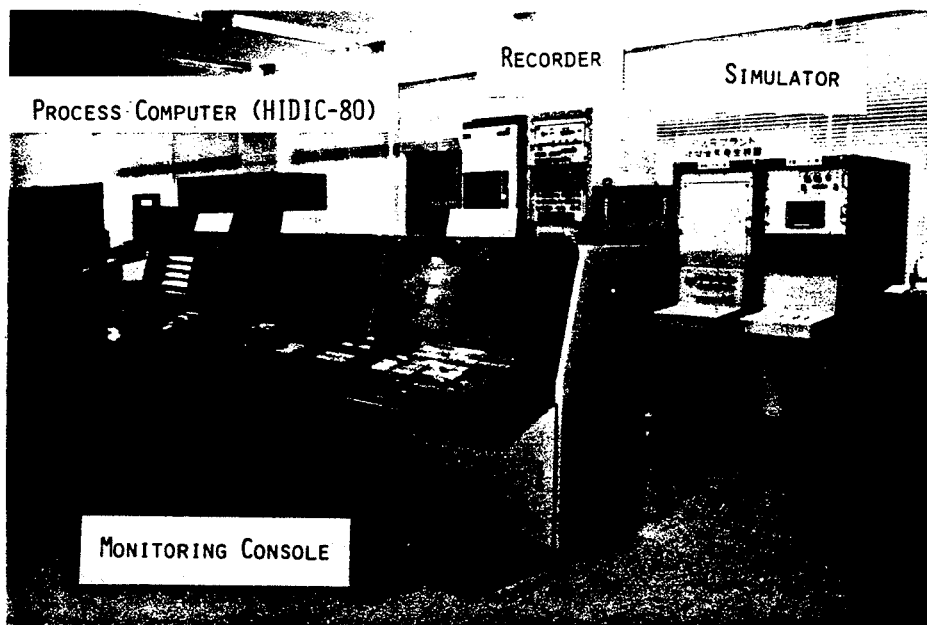
Photo. 2 Computer Based Plant Operation Monitoring Console
