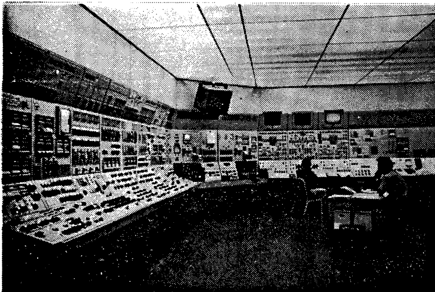
FIGURE 9 Example 2 of Control Room Layout Pickering 'A' (Station 2)
