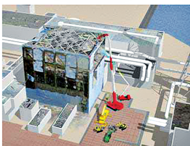
Debris removal from the upper part of reactor building
