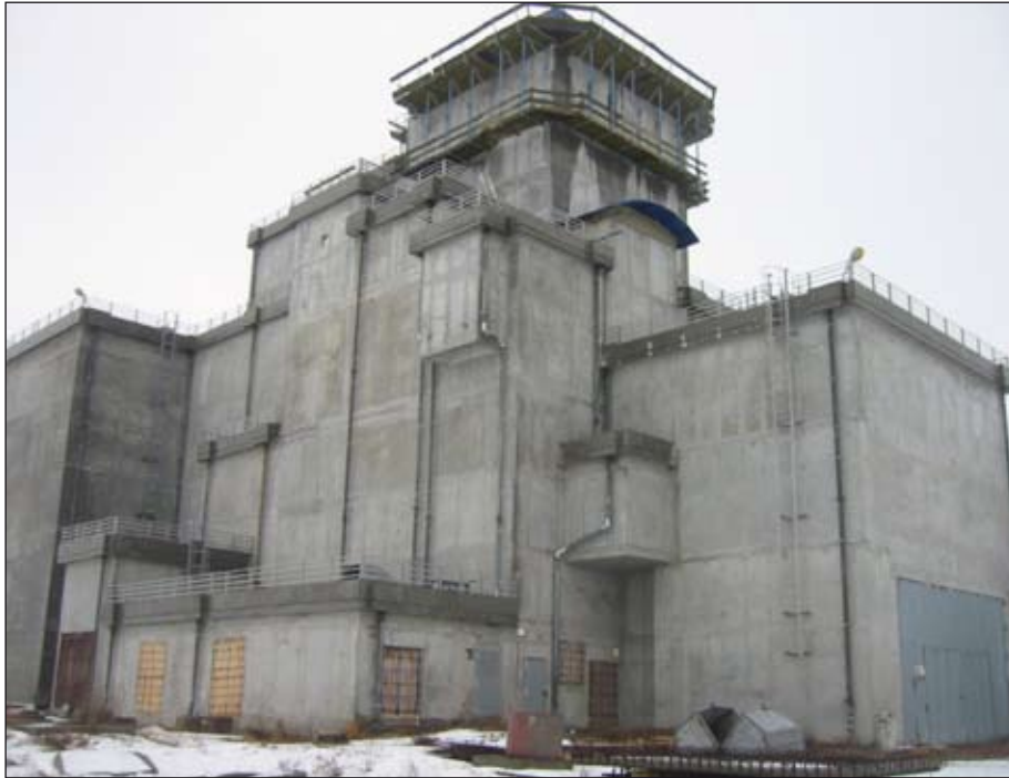
Fig. 8. Process- and conditioning building of the intermediate storage facility – ISF-2.
