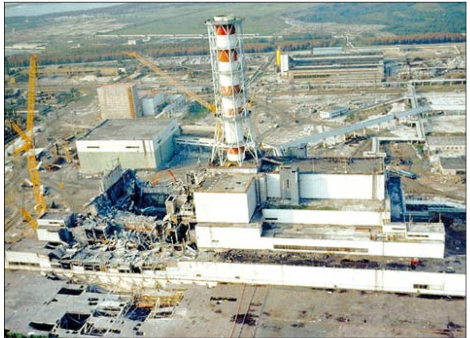
Fig. 5. The destroyed Unit 4 (left) and Unit 3 (right) of the Chernobyl nuclear power plant.
