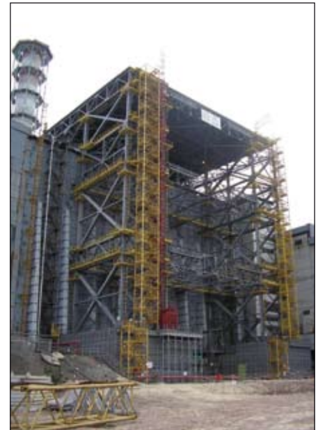
Fig. 3. Stabilisation measures at the Western wall of the sarcophagus.
