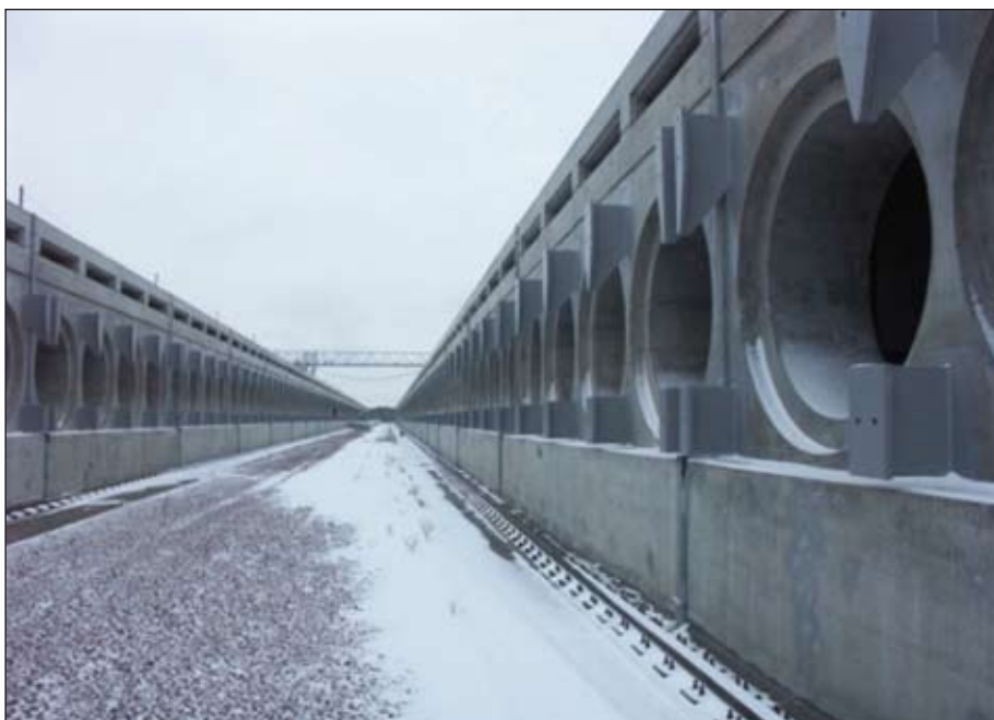
Fig. 9. Storage modules of the intermediate storage facility ISF-2.
