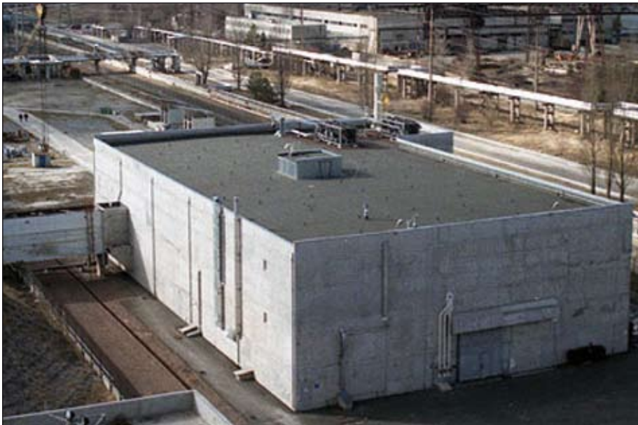
Fig. 7. Treatment plant for liquid low- and medium-level waste – LRTP.
