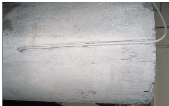
c. installed cable
