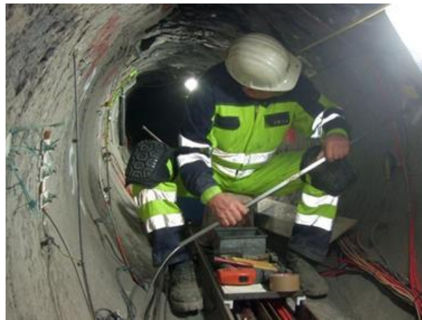
Fig. 4.7 Installation of GRS minipiezometers in the microtunnel
