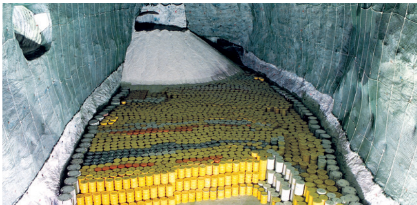
Drums containing radioactive waste in the Morsleben (ERAM) repository
