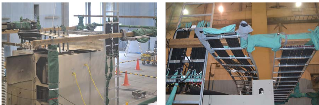
Figure 8 Damage of equipment observed in Phase-2 (Test No. 5-1)
