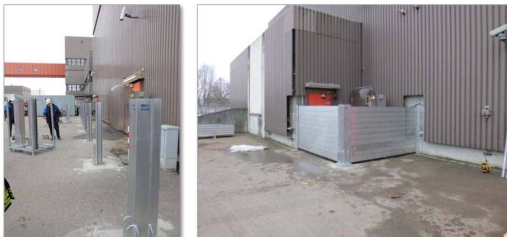
Figure 10 Flooding barrier wall
