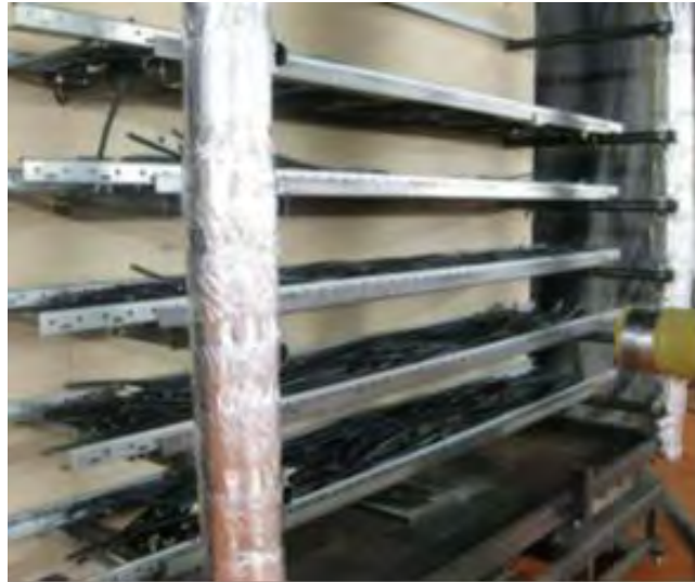
Figure 1 The five horizontal cable tray device used for the CFSS fire tests
