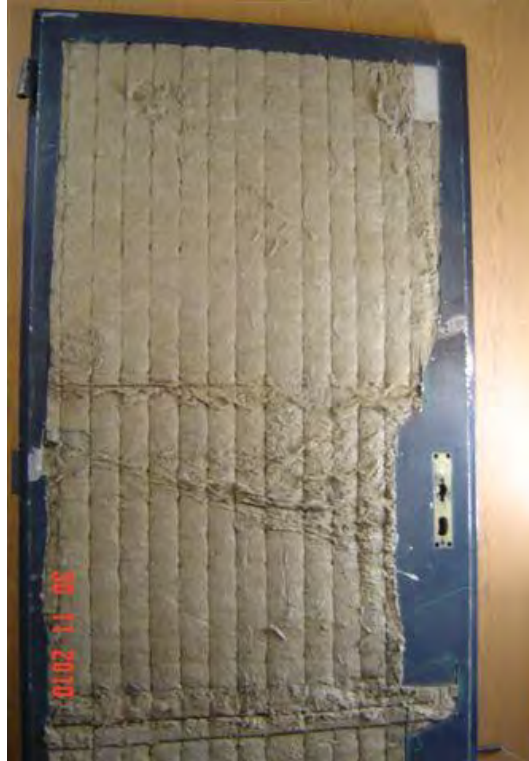
Figure 3 Example of a fire door according to the old DIN standard being cut open after removal from the plant showing no deterioration of the insulation
