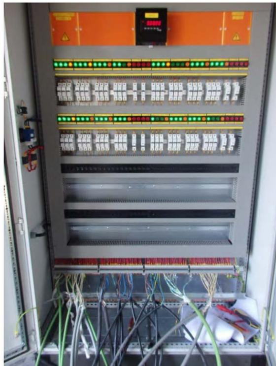
**Figure 4** Circuit control rack of the fire test
