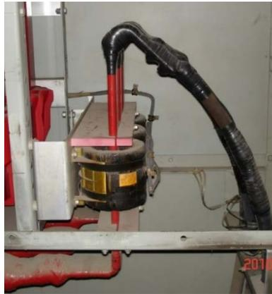
**Figure 1** Window-type CTs shown with bus bar as primary circuit [3]
