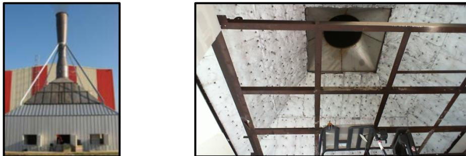
**Figure 1** Hood (outside and inside top views) gathered the smoke by natural ventilation
